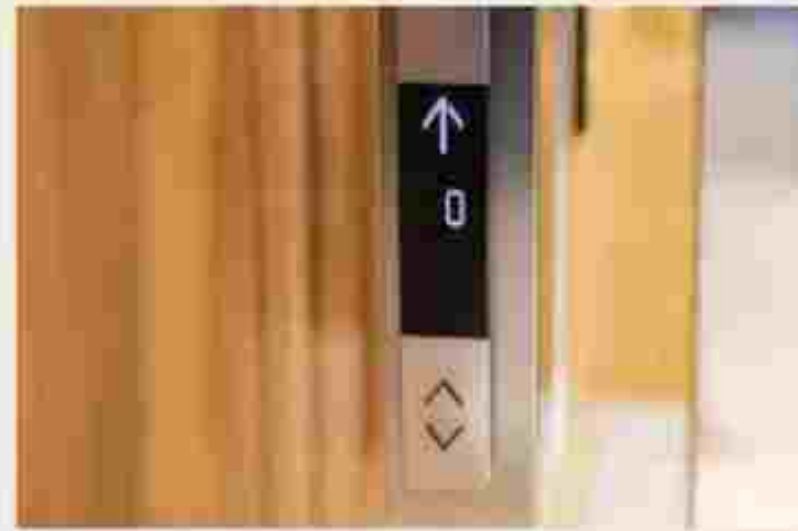
Elevator in each mansion
