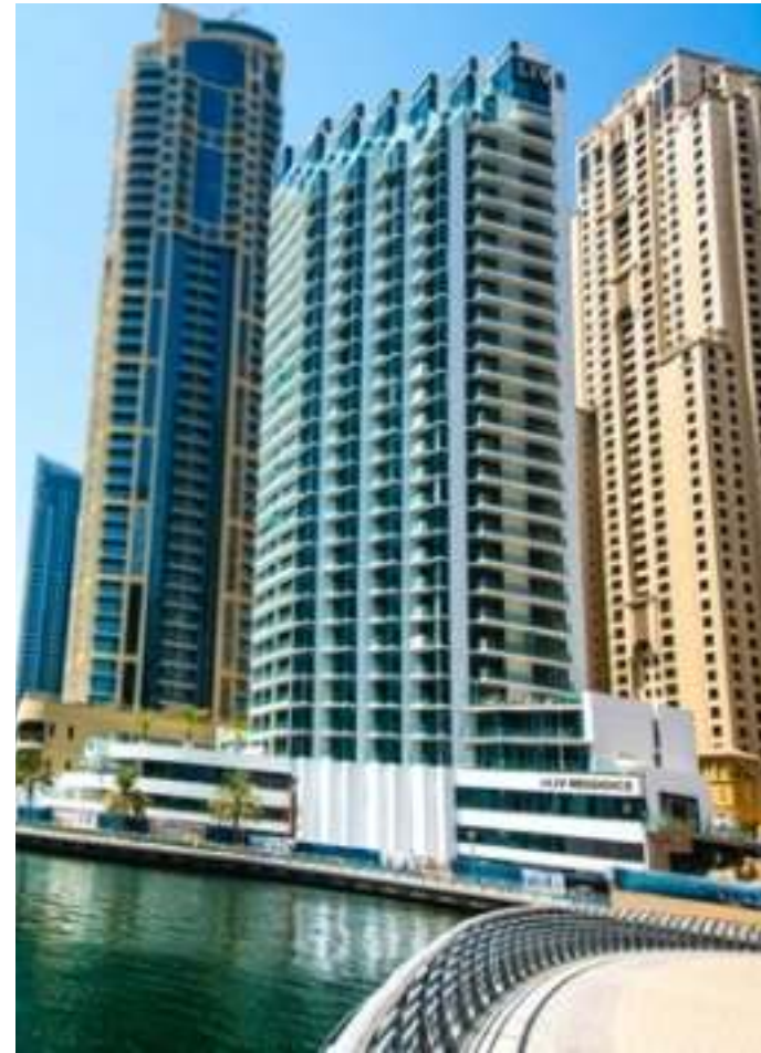
LIV Residence COMPLETED & HANDED OVER
