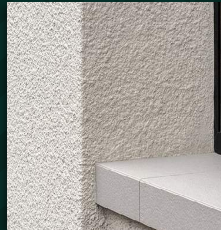
3 - PLASTER WITH PAINT
