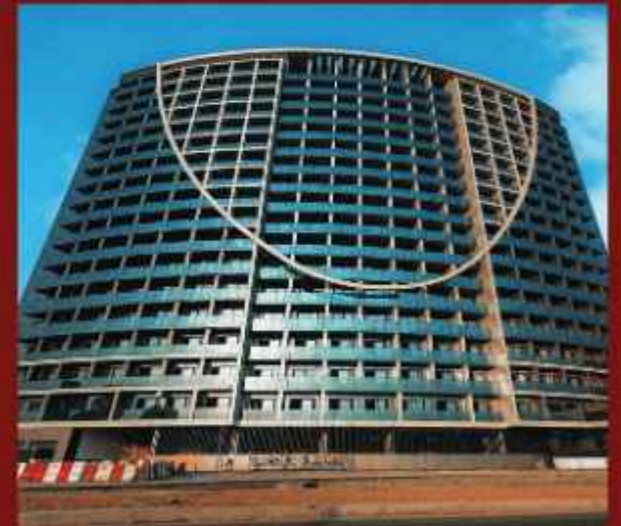
The V Tower
