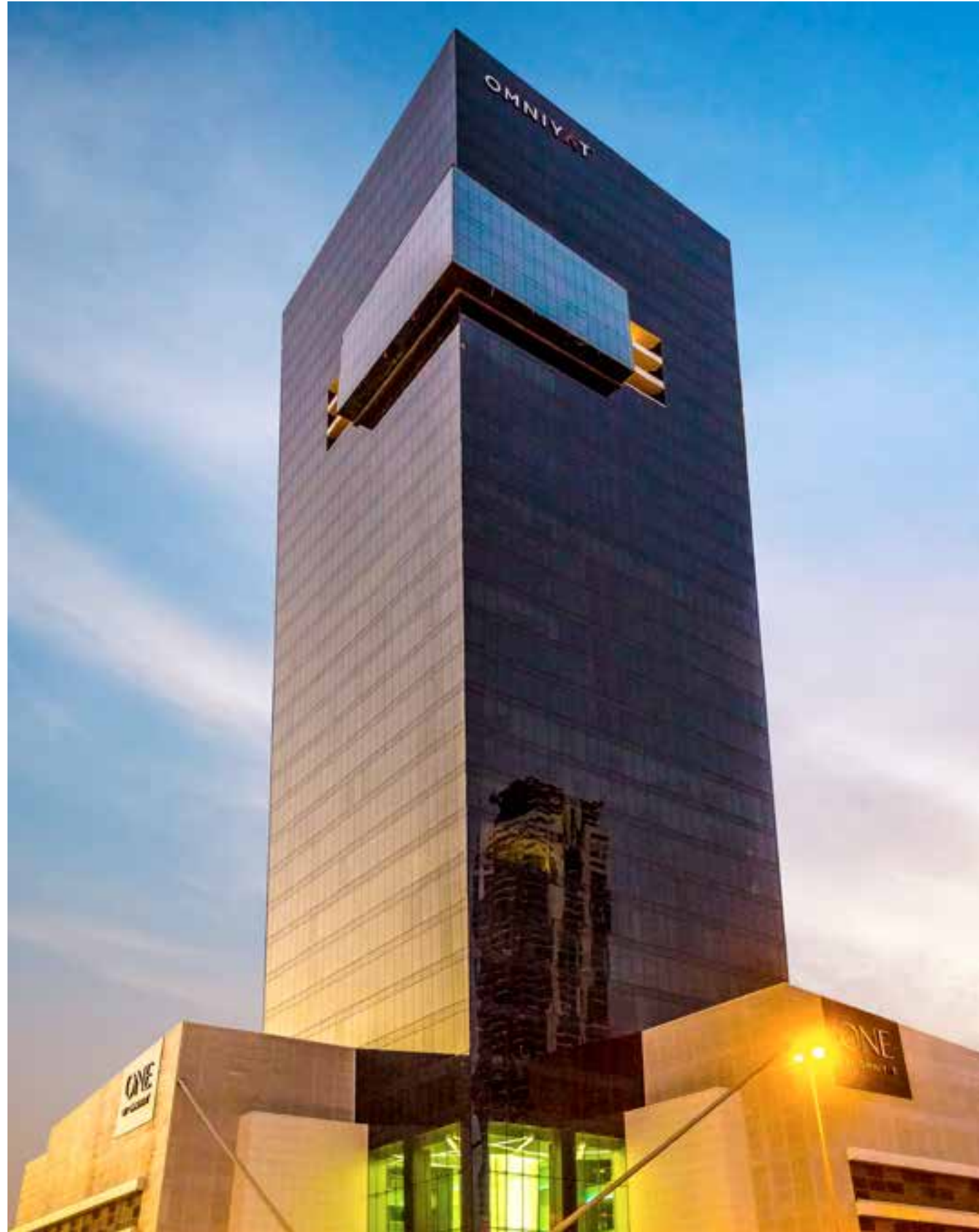
ABOVE: ONE BY OMNIYAT, OMNIYAT'S NEW SIGNATURE COMMERCIAL TOWER, LOCATED JUST OFF SHEIKH ZAYED ROAD AT THE ENTRANCE TO THE BURJ KHALIFA DISTRICT.
